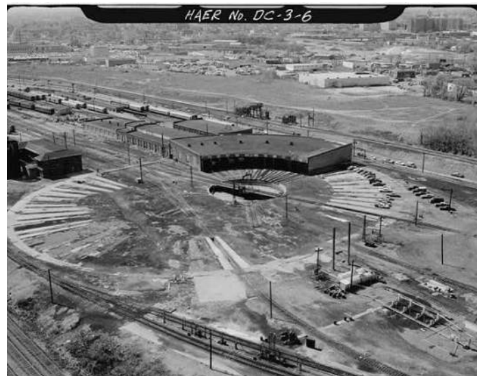
Aerial Photograph, Ivy City Roundhouse, 1977
